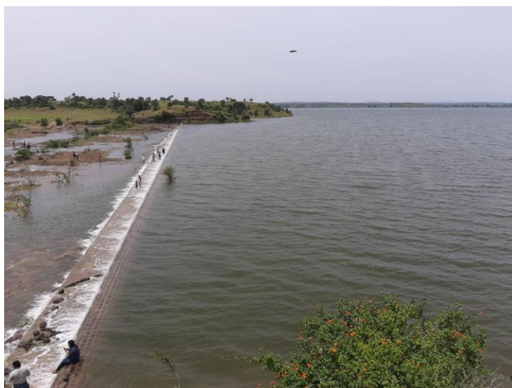
A view of Khelna reservoir.
